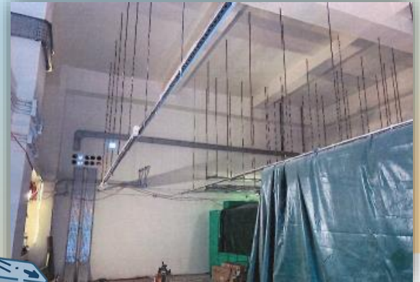
Electrical Installation at LV Main Switch Room 總制房電力安裝
